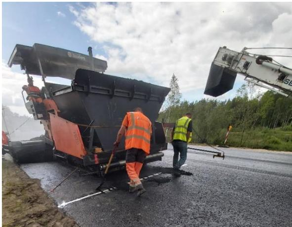
**Fig.1.** FBG strain and temperature sensors integration into road pavement
